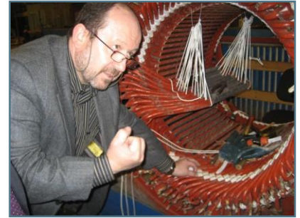
Specific electrical machine inspection
